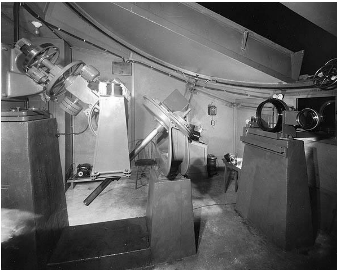
Fig. 35. This is a composite image from two photos of the siderostat system. Because the shots were taken from two different positions, there is a discontinuity of perspective from right to left across the illustration. The “stationary” 15-inch objective and the finder objective appear at right. The large objective is stationary only in east-west and top-to-bottom senses; it can be moved on rails in the north-south direction for focus. The pier for the equatorial mount is at the left edge of the picture and the polar axle can be seen clearly. The sliding-bearing linkage of the equatorial mount to the altazimuth one is invisible behind a 5-inch camera and the 25-inch flat appears very nearly edge-on and cannot be seen. The finder objective and its feeder flat were removed at a later time. The paint finish was the same as that on the reflector. In this view of the hardware room, the roof shutters are open.
