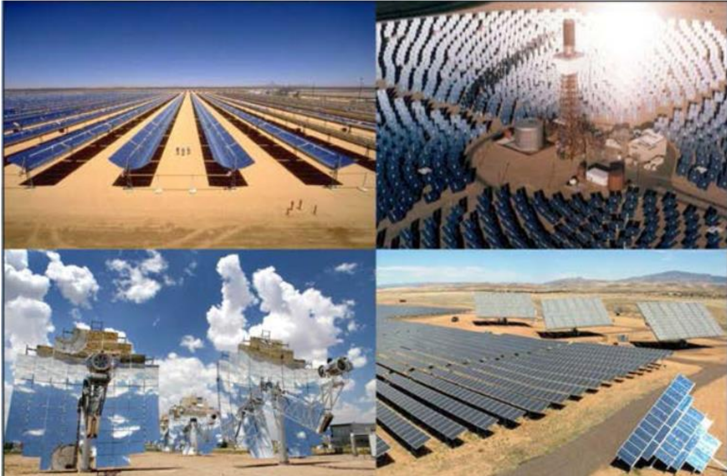
Typical Solar Fields for Various Technology Types (clockwise from upper left): Solar Parabolic Trough (Source: NREL/SR-550-32282), Solar Power Tower (Credit: Sandia National Laboratories. Source: NREL), Photovoltaic (Credit: Arizona Public Service. Source: NREL), and Dish Engine (Credit: R. Montoya. Source: Sandia National Laboratories).
